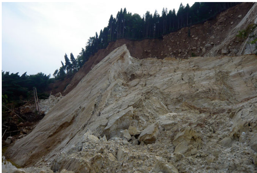
Fig. 10.33 Sampling site at a lower part of Aratozawa landslide
