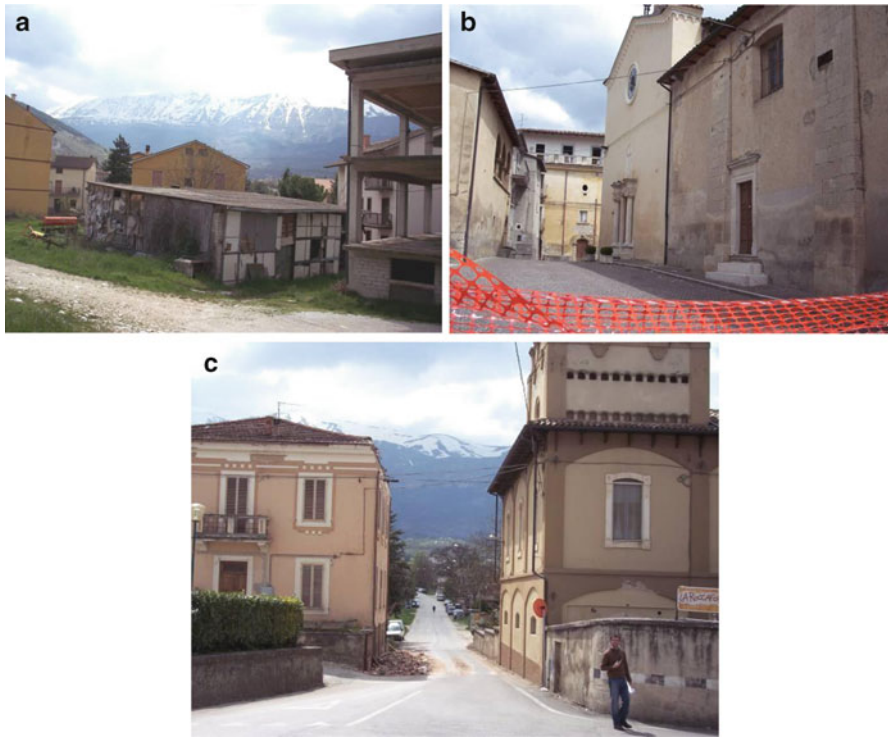
Fig. 1.47 Monticchio : (a) D0 damage level on different building structures; (b) D0 damage on monumental masonry buildings; (c) D1 damage (fall of the cornice) on a masonry building
