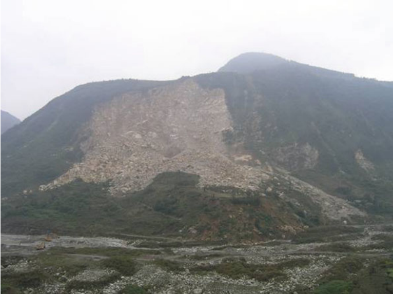
Fig. 2.7 Surface failures near Yingxiu
