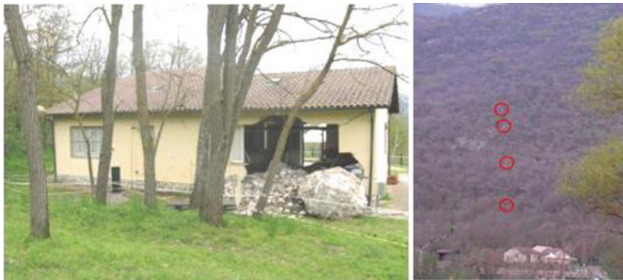
Fig. 1.57 Block detached from a rock cliff above the Stiffe Caves (left). Impact marks (on the right) individuated by Scott Kieffer and Edward Button (GEER Working Group 2009)
