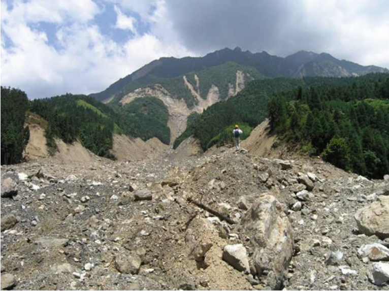
Fig. 2.3 Slope failure at Xiejadian site in Pengzhou city
