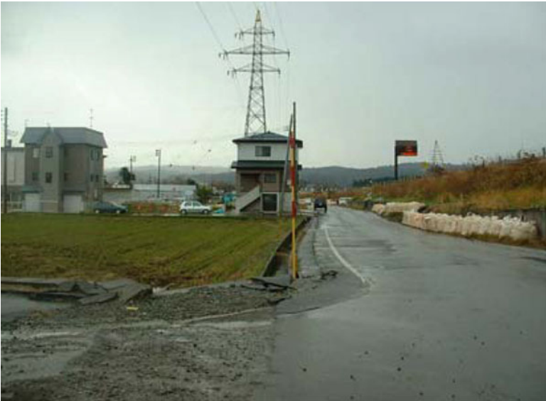
Photo 9.9 Moved ground adjacent to C-Box Ojiya 2
