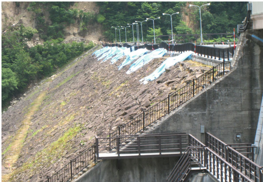
Fig. 10.8 Settlement features of the dam crest indicating presence of hidden pillars, Ishibuchi dam (Looking over the right abutment)
