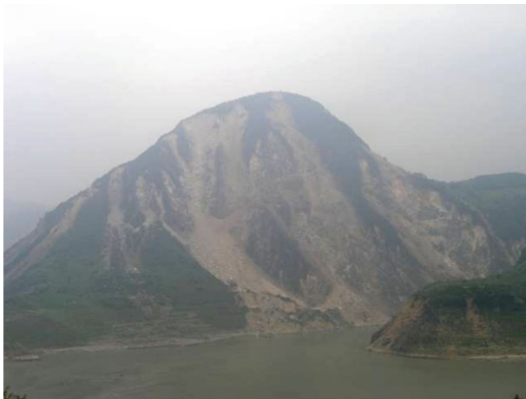
Fig. 2.10 Surface failure from top of mountain on the Zipingpu dam reservoir
