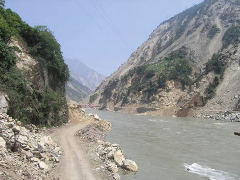
Fig. 2.8 Continuous failures in Minjiang valley slope in Yingxiu
