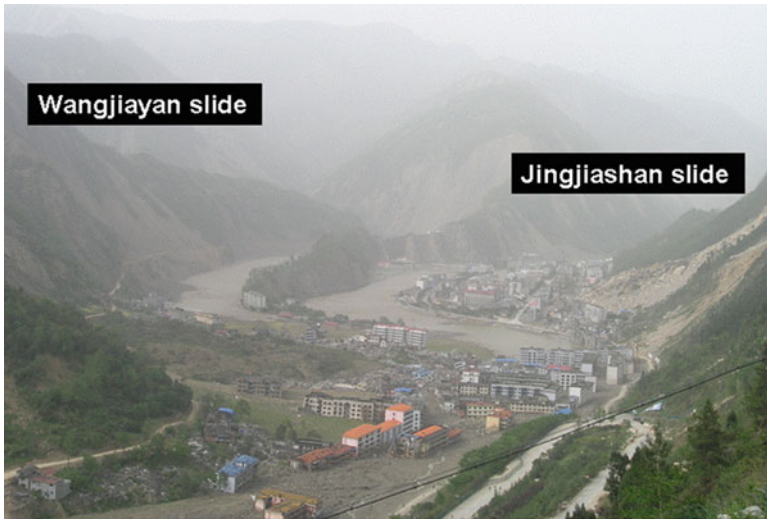
Fig. 2.21 Post-earthquake expansion of Wangjiayan slide in Kushan town of Beichuan county
