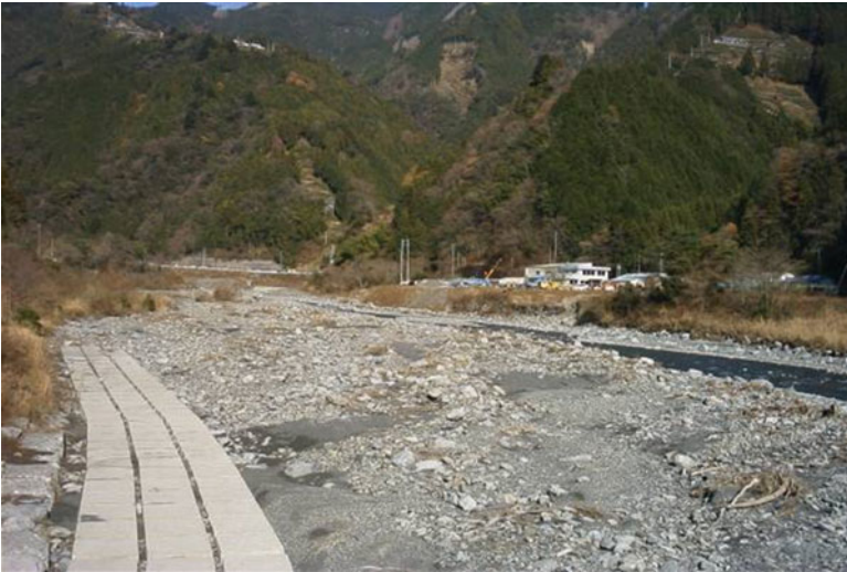
Fig. 2.20 Abe river channel filled with frequent debris flow
