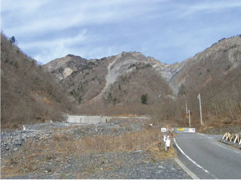
Fig. 2.19 Ohya landslide of Abe river in Japan
