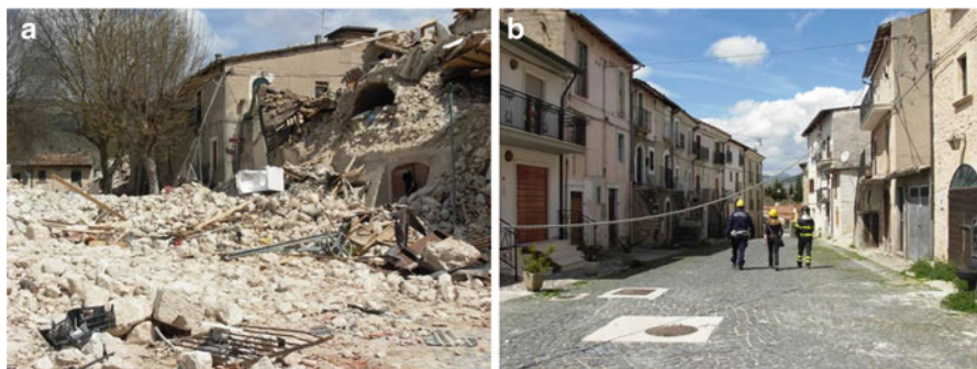
Fig. 1.50 Castelnuovo: (a) collapse (D5) of old masonry buildings on the hilltop; (b) limited damage (D1-D2) to masonry buildings at the toe of the hill
