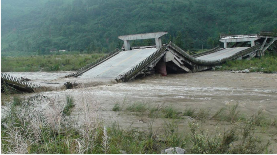
Fig. 2.24 Collapse of Xiaoyudong bridge (Photograph by Huang Dong)
