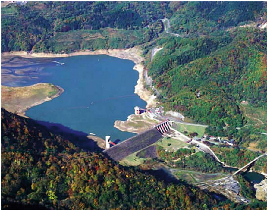
Fig. 10.3 Bird-eye view of Ishibuchi rockfill dam (From the office of Ishibuchi dam)
