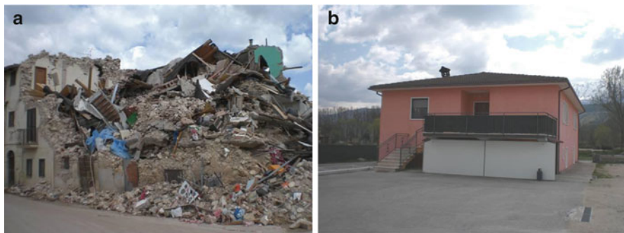
Fig. 1.46 Onna: (a) D5 damage level on masonry building structures; (b) D0 damage on an r.c. building (except for the tilting of the chimney)
