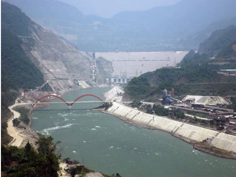
Fig. 2.30 Successful behaviour of Zipingpu dam near Dujiangyan. (Photograph from www.chinawater.com.cn )
