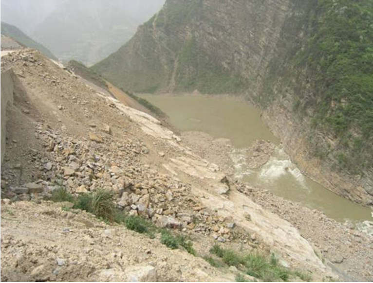
Fig. 2.11 Different extent of slope damage due to different geological settings
