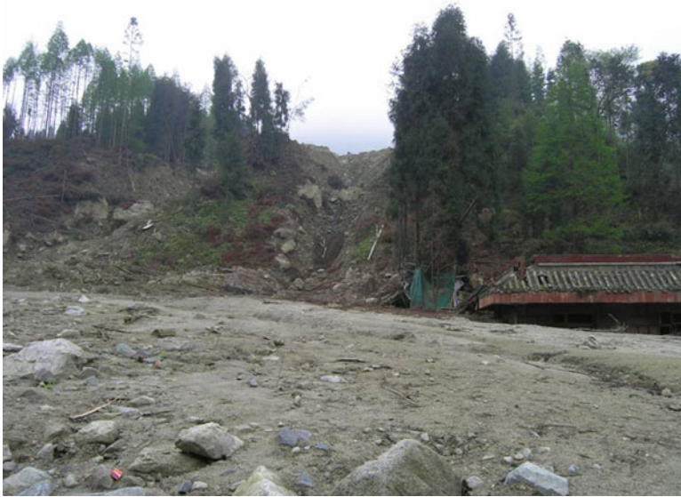
Fig. 2.23 Rainfall-induced debris flow in Yinchanggou
