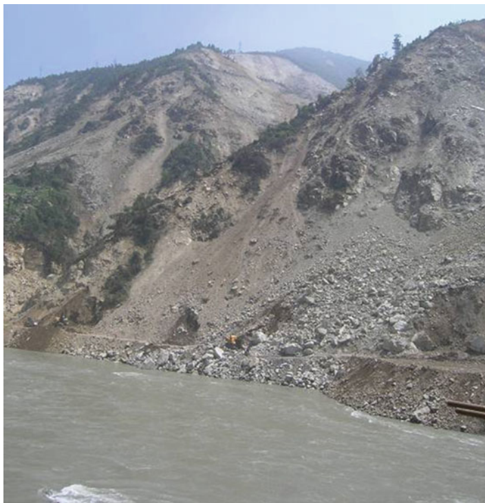
Fig. 2.9 Road destroyed by surface failure near Yingxiu
